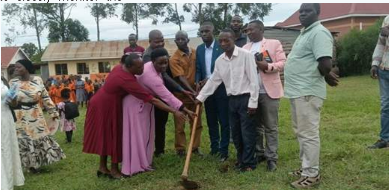
Kalungu District officials and the technical team officially launching the construction of a two-classroom block with an office at Kapeere Memorial School in Lukaya on 5th March 2026.
