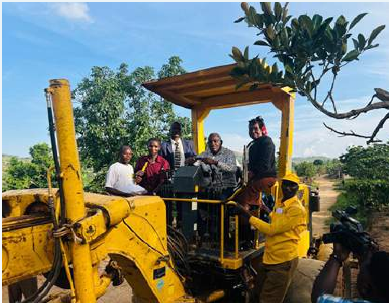
RDC Emmy Kateera, accompanied by other district officials, launching the rehabilitation of the Bwingana-Kawule-Kagaga Road in Malongo Sub county on 9th March 2026.
