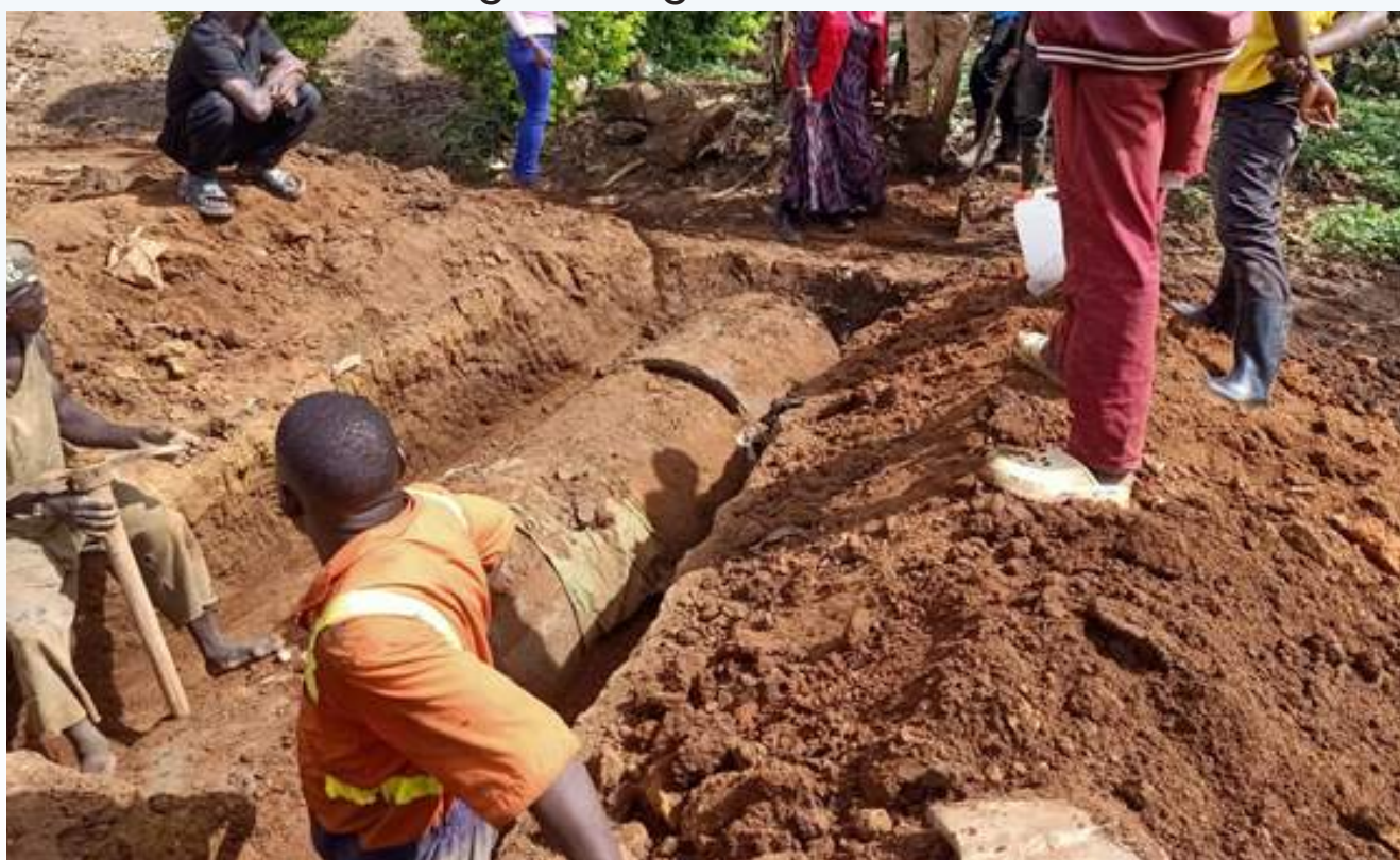
Butambala District Woman MP Hon. Aisha Kabanda Nalule, with some district leaders inspecting progress on work done at Kasansala road in Ngando sub county on 3rd March 2026.
