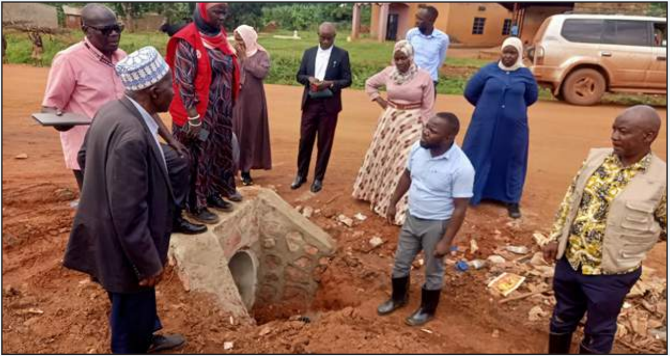
Butambala District Woman MP Hon. Aisha Kabanda Nalule, with some district leaders inspecting progress on work done at Bulu Bugobango road in Bulu sub county on 3rd March 2026.
